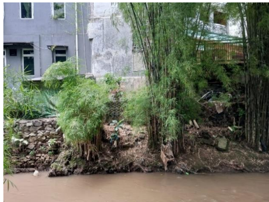
Figure 4. Residents' settlements on the banks of the Krukut River
