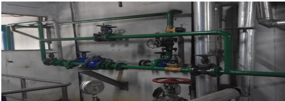
Figure 3. Installation of Pipes and Fittings after the Modification
