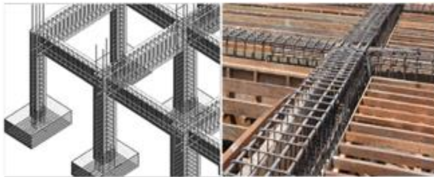
Figure 1. Beam with vertical stirrup reinforcement
