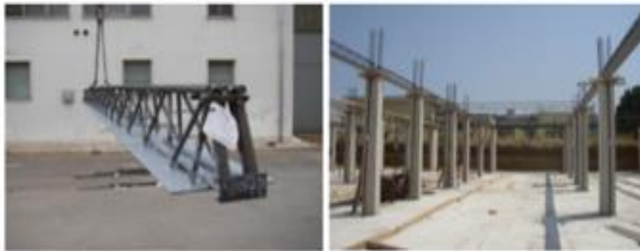
Figure 2. Concrete beam reinforcement frame structure
