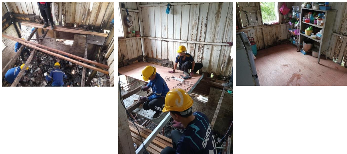
Figure 6. The Process of Substituting the Kitchen Floor
