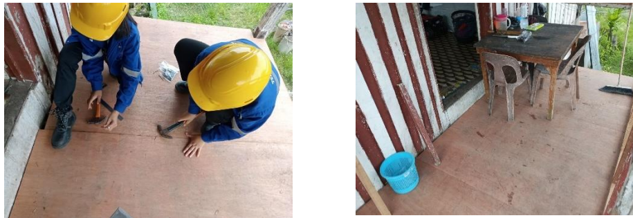
Figure 7. The Process of Substituting the Porch Floor
