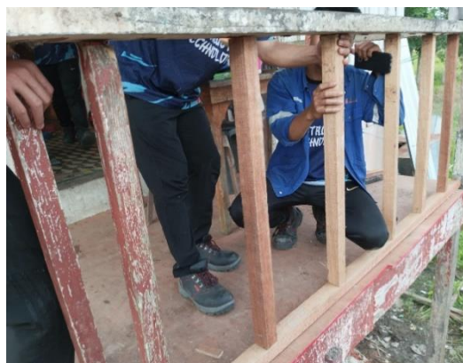
Figure 9. The Replacement of the Railings at the Porch
