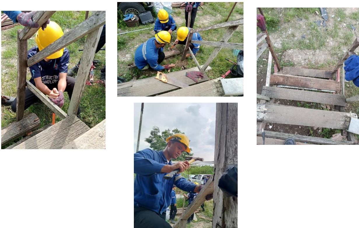
Figure 8. The Reinforcement of the Stairs
