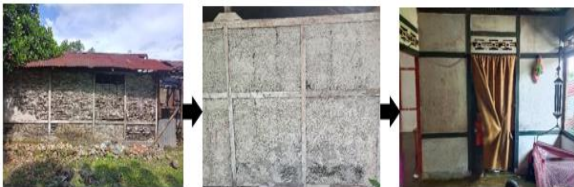
Figure 2. Example of a button house with walls of woven bamboo and plastered with cement so that the bonding power is strong and the house does not collapse or crack easily
